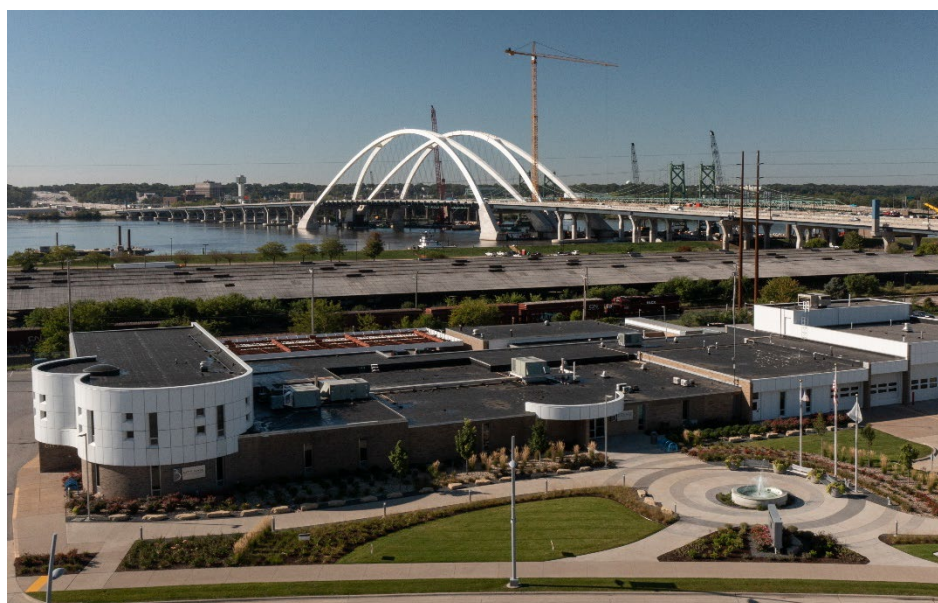
City Hall with I-74 Bridge construction in the background
